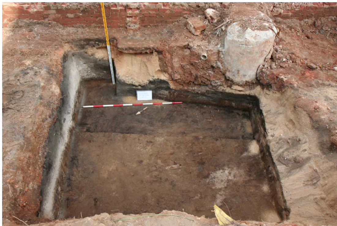
Figure 19: VCH 005 with concrete test pile. Coarse marine sand is visible in centre above clipboard
