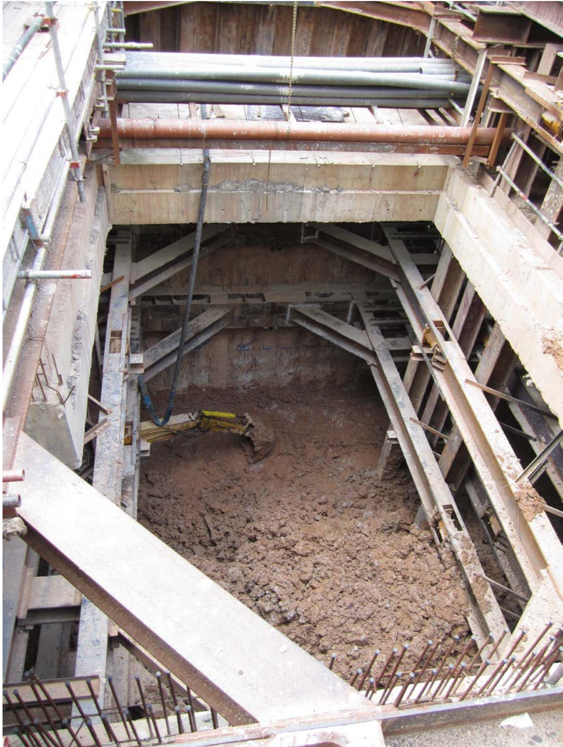
Figure 27: Subterranean complex for mechanical and engineering services
