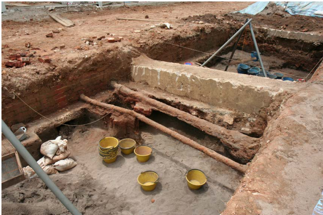
Figure 22: VCH 008 looking south, revealed numerous modern utilities
