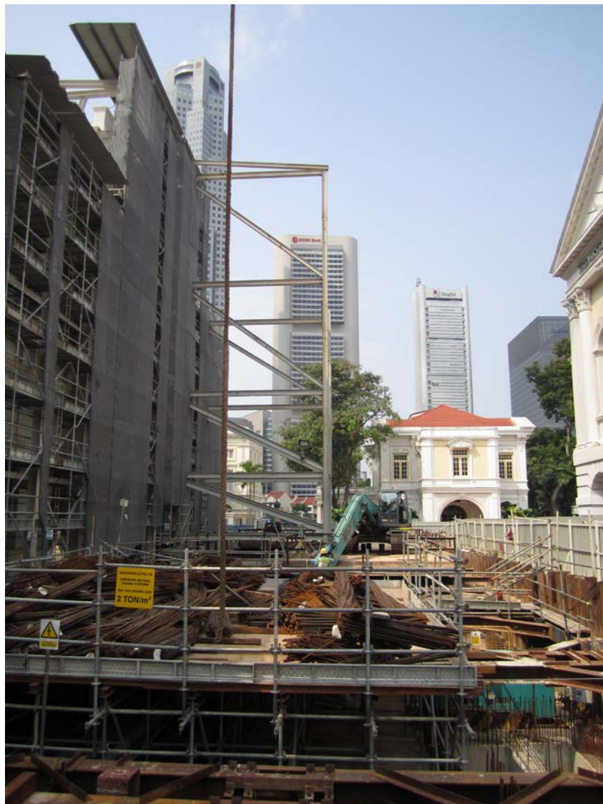
Figure 26: Construction of subterranean complex for mechanical and engineering services
